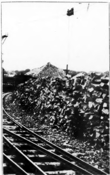
Broken Stone Stored Along Tracks
